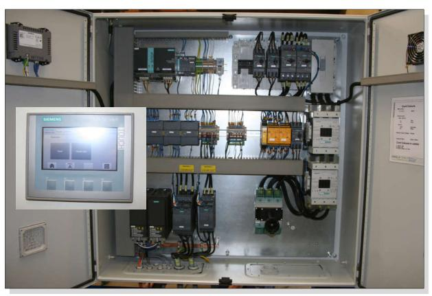
The control cabinet. Insert: The HMI-unit.
