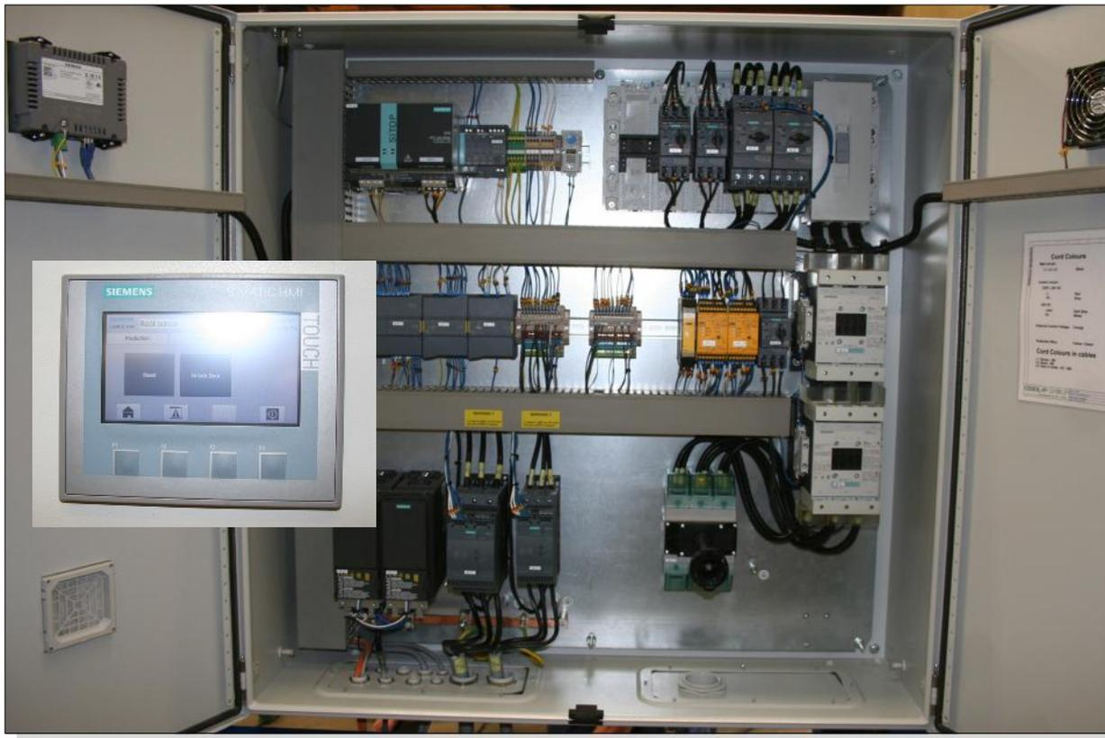
The control cabinet. Insert : The HMI-unit.
