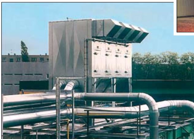
Filter system for 240,000 m<sup>3</sup>/h for window factory in Scotland with silo system for storage of chips before combustion.
