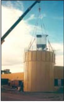
Modular silos in sizes from 10-500 m<sup>3</sup> in diameter 2-7 metres with pitched roof for cyclone or flat roof for filter system.
